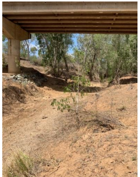
Plate 3-11 Deep Creek Dry Reach [October 2019] / Upstream of Bruce Highway Bridge
